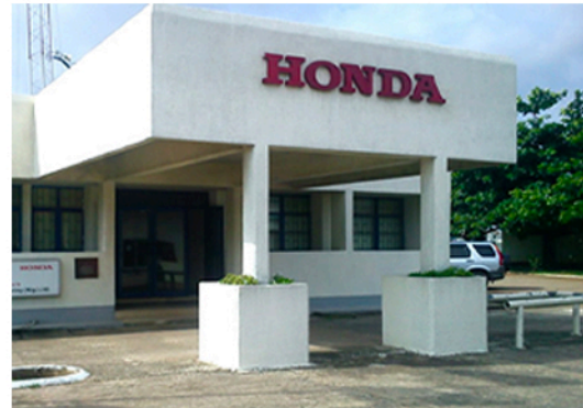
Honda Manufacturing Company Ota/Idiroko Expressway
